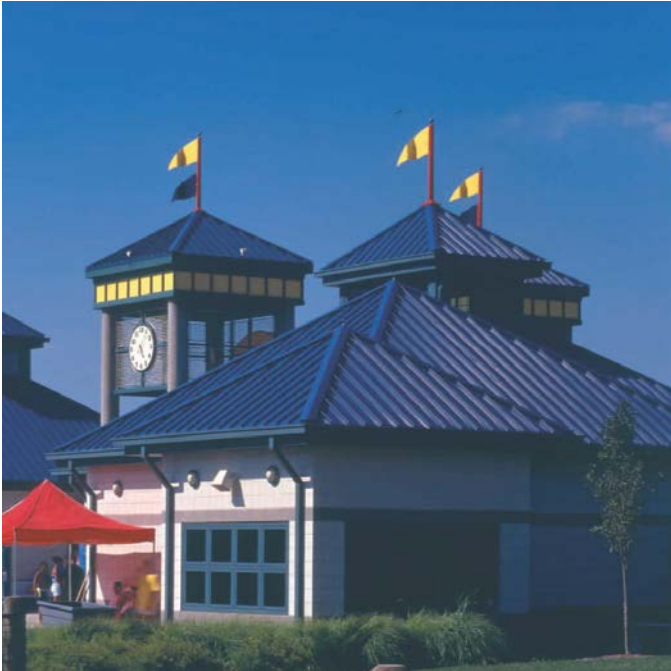
▲The Sycamore Trails Aquatic Center, Miamisburg, Ohio, features a Snap-Clad (Peterson Aluminum) roof in interstate blue with teal-colored trim.
